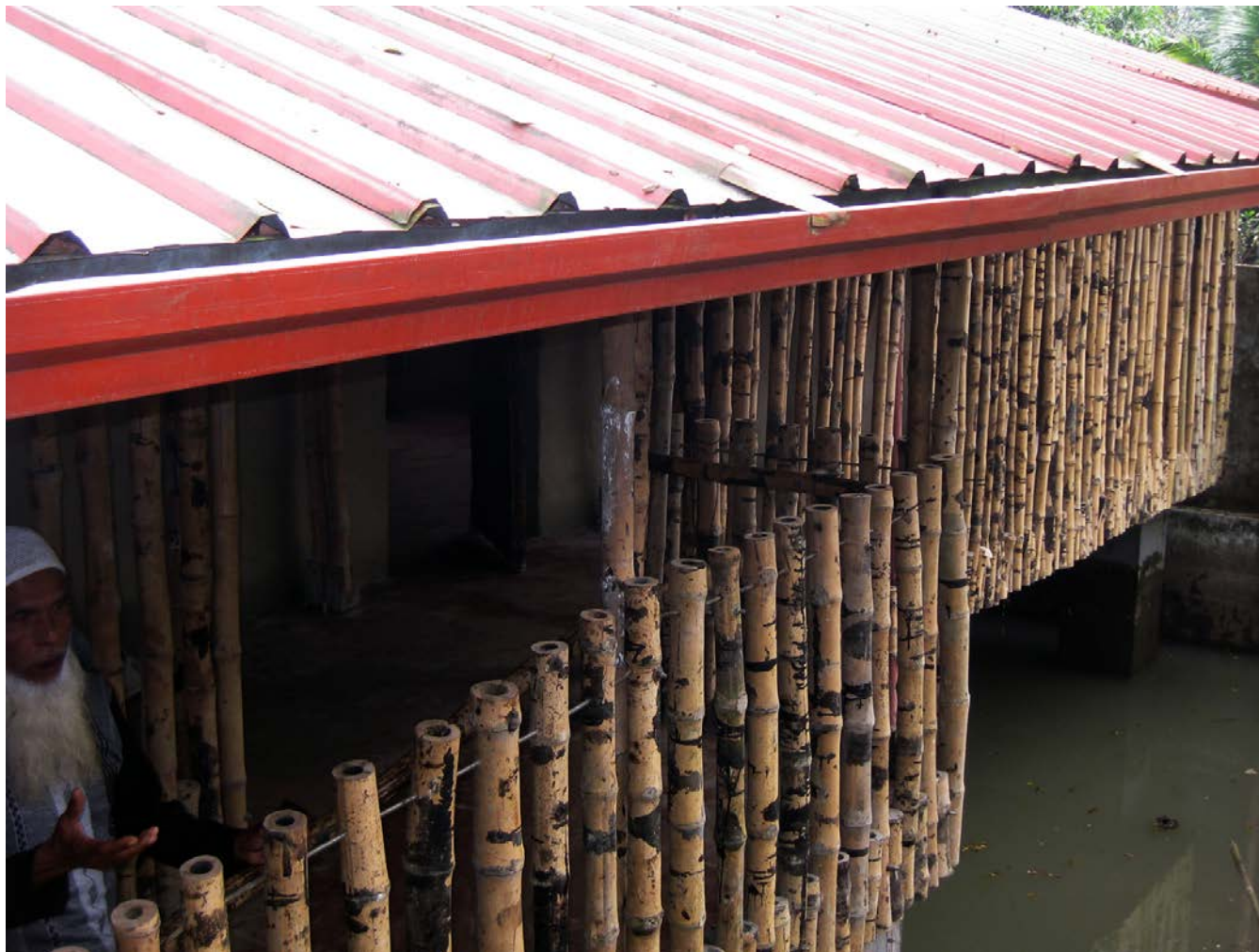
Fig. 46 Perforated bamboo wall veranda, where the effects of the evaporative cooling (from the pond below) is felt
