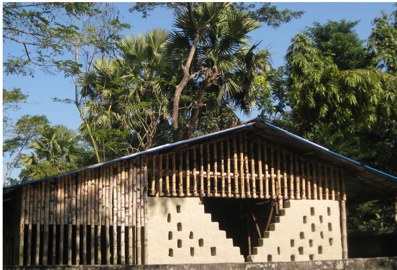
Fig. 4 Side elevation of building, showing handmade bricks and bamboo construction
