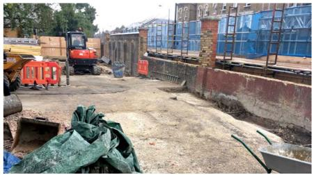
Fig. 32 Eleanor Palmer Science Lab, at the start of the build showing scaffold supporting the boundary wall from collapse
