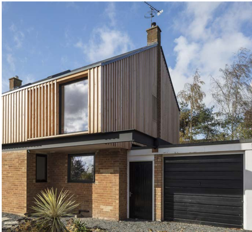
Fig. 3 Phase 1 house. Rear view showing timber overcladding at first floor and horizontal characterisation of a design intended to improve on the existing building's 1970s characteristics Photo: Matt Chisnall
