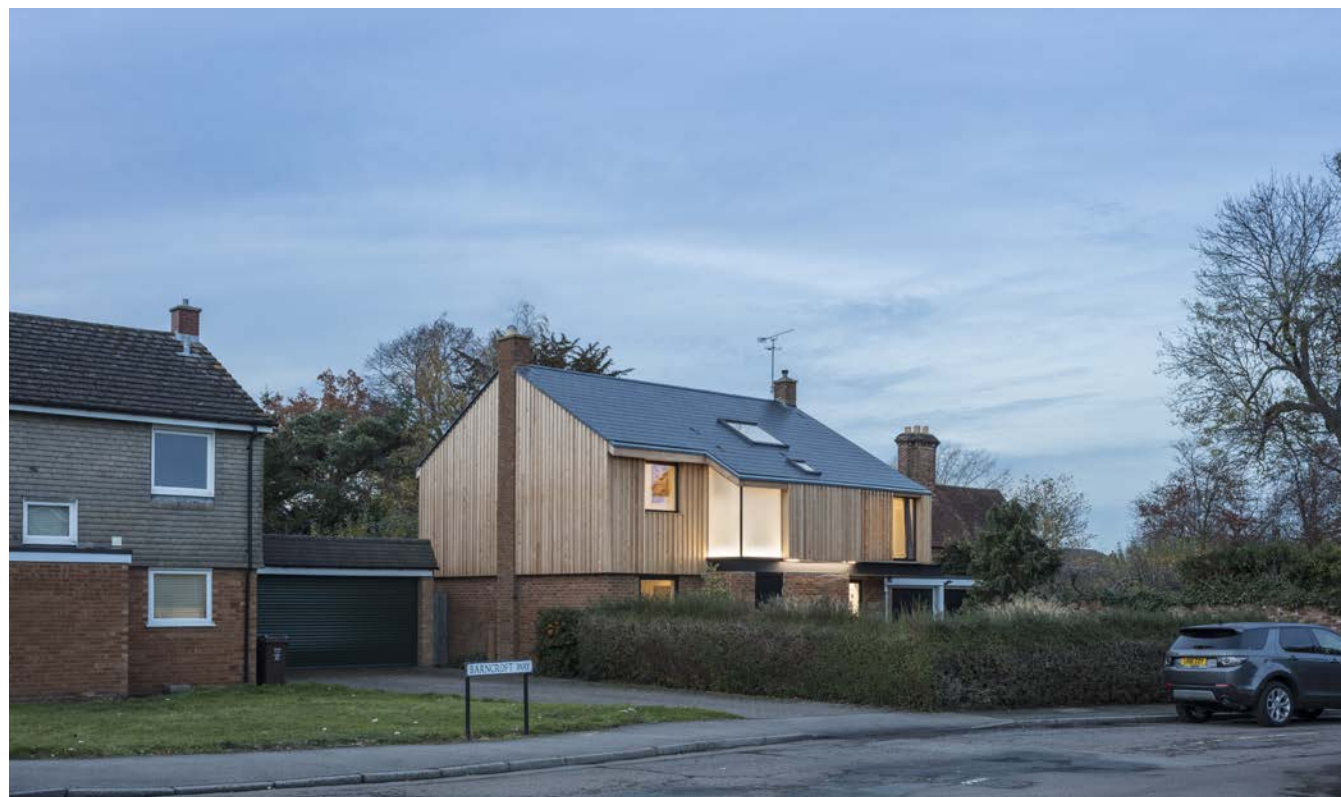
Fig. 51 St Albans house exterior: The house is warmer and lighter than previously. The larch overcladding refers back to the site's rural history Photo: Matt Chisnall
