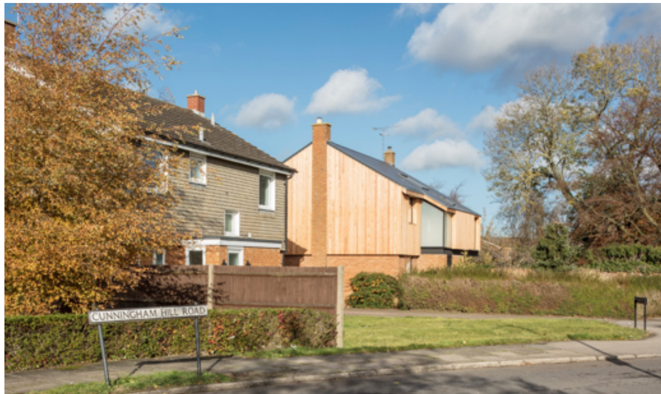
Fig. 64 View along Barncroft Way showing the retrofitted house compared with its original neighbour Photo: Matt Chisnall
