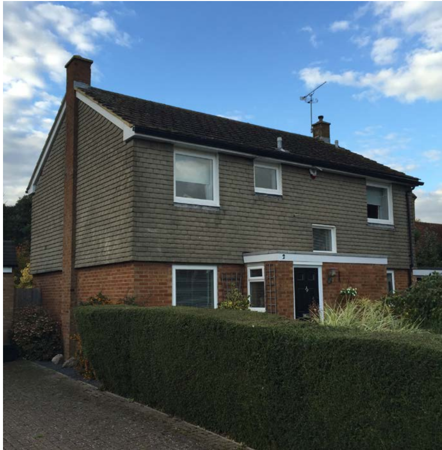
Fig. 5 Original house showing classic 1970s characteristics which were deployed in new ways in the refurbishment, including differentiation of first floor and strong horizontal characteristics
