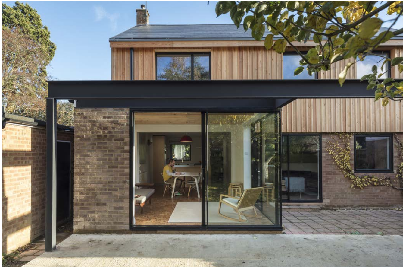
Fig. 3 Phase 1 house. Rear view showing timber overcladding at first floor and horizontal characterisation of a design intended to improve on the existing building's 1970s characteristics Photo: Matt Chisnall
