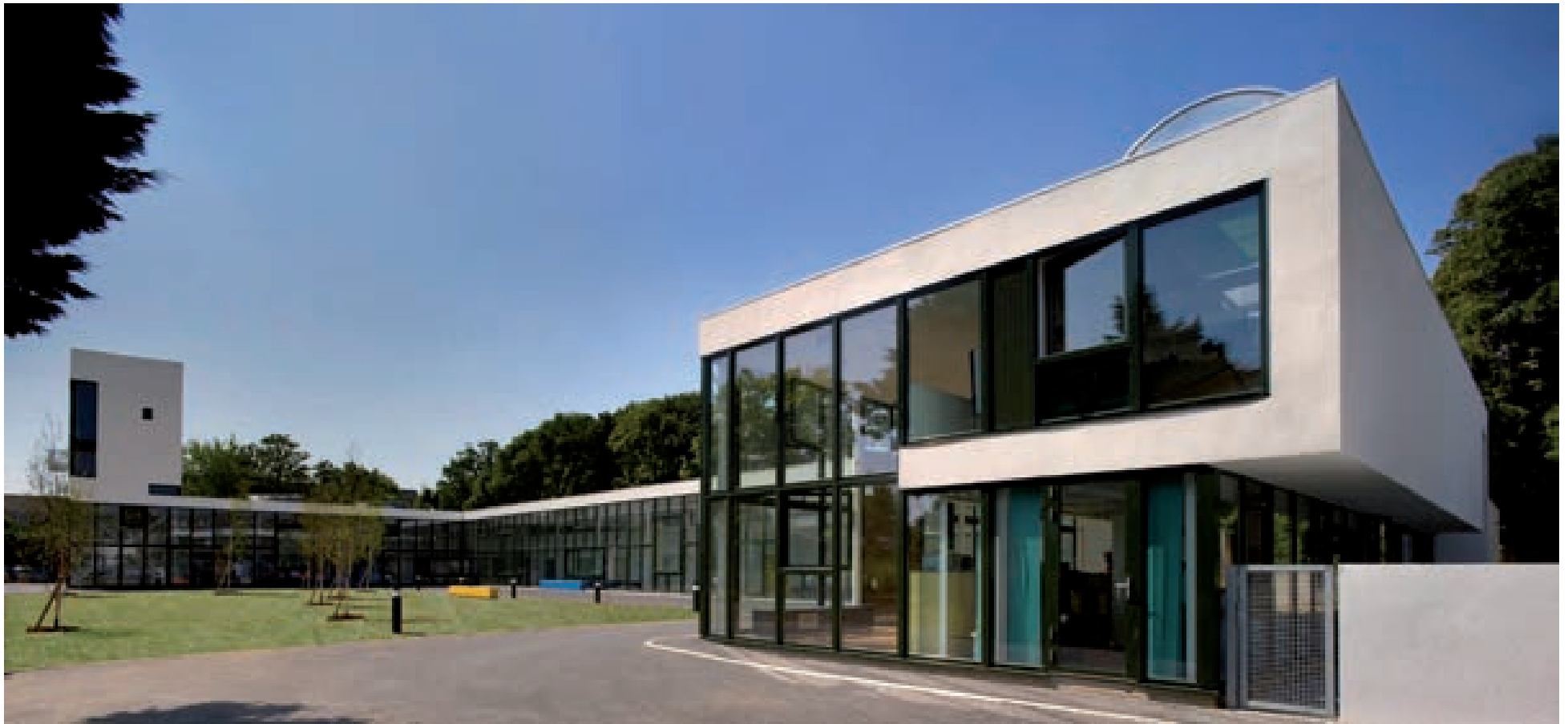
Fig. 14. Spring Gardens: View from entrance, photograph Morley Von Sternberg
