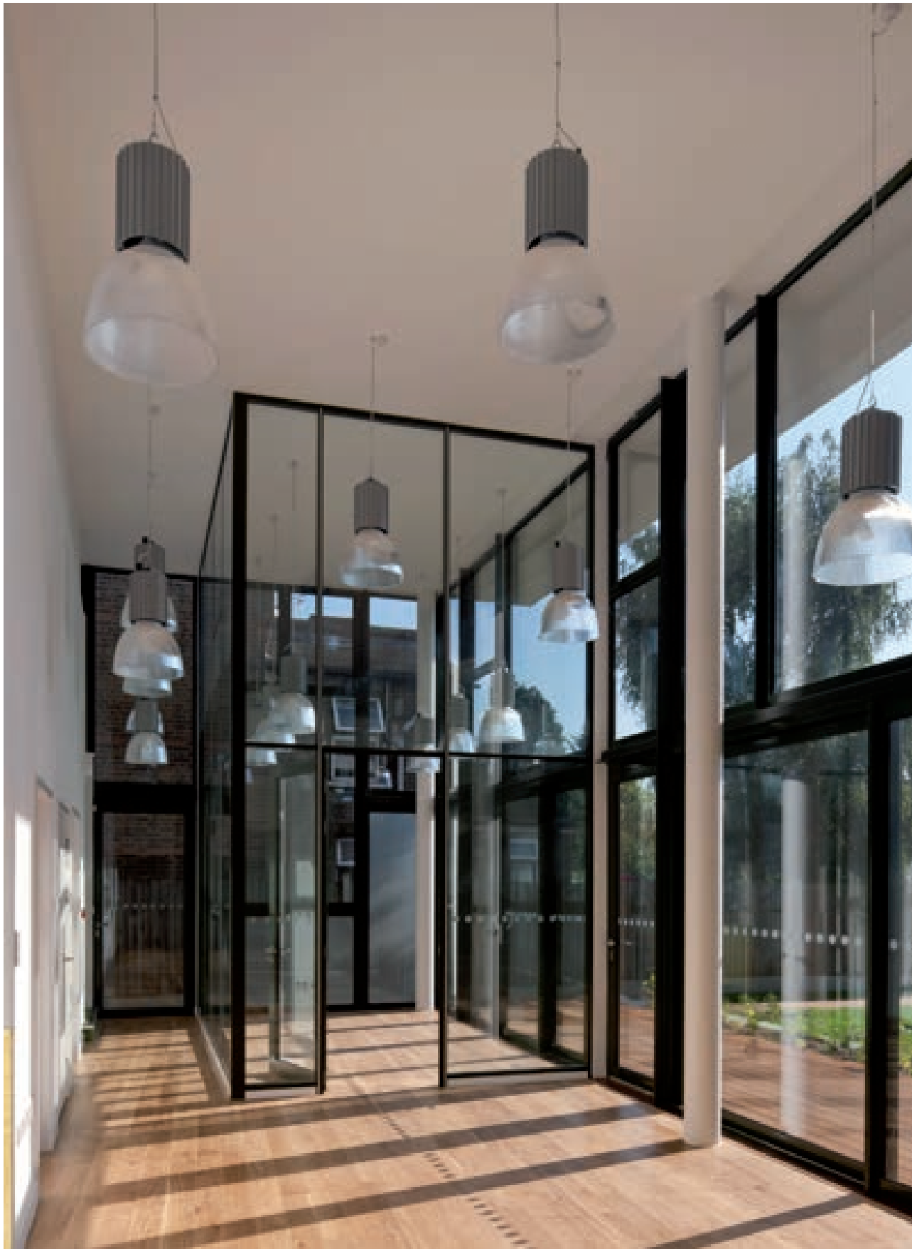
Fig.37. Welcome Centre: Glazed lobby, entrance lock, photograph Morley Von Sternberg
