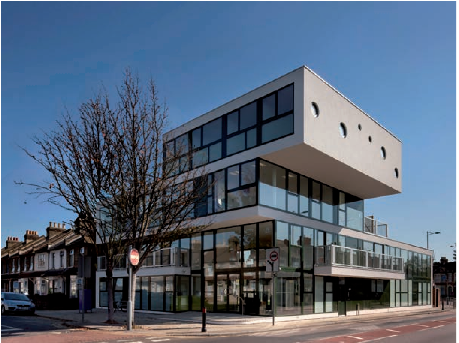
Fig.35. Welcome Centre: View from corner of St. Mary's Road and Green Lane, photograph Morley Von Sternberg
