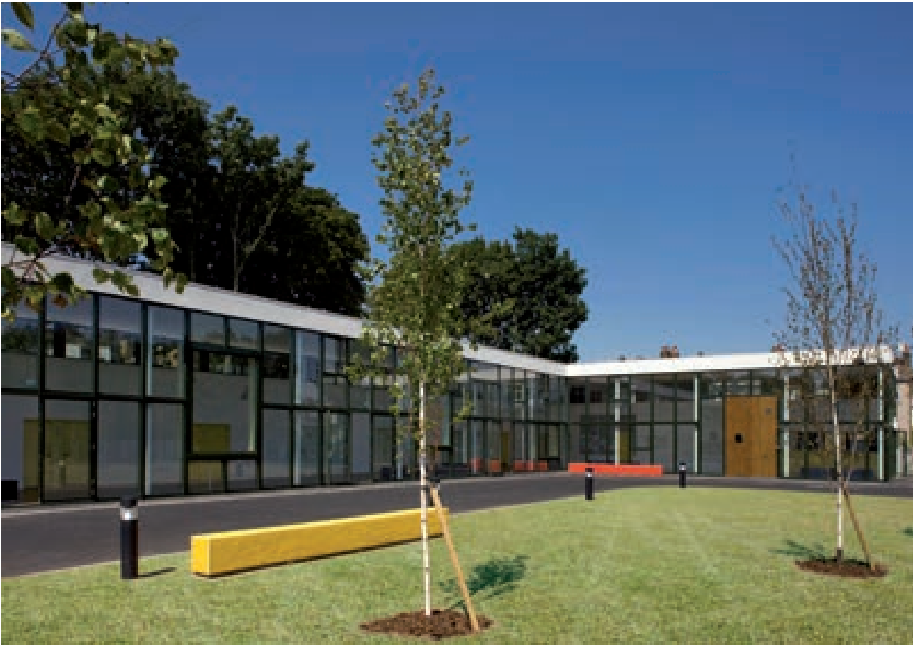
Fig.15. Spring Gardens: View towards entrance, photograph Morley Von Sternberg
