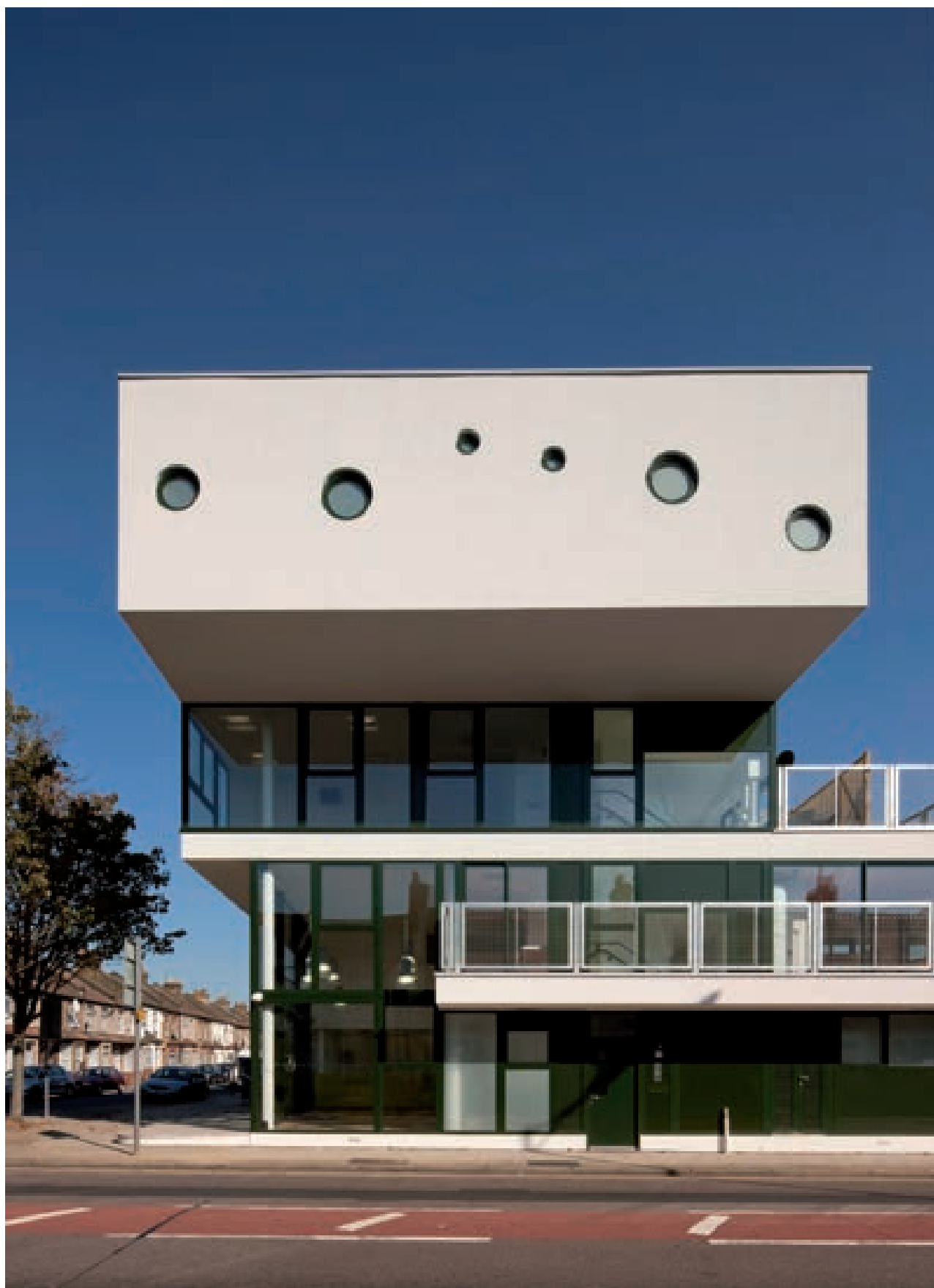
Fig.36. Welcome Centre: View from Green Lane, detail, photograph Morley Von Sternberg.
