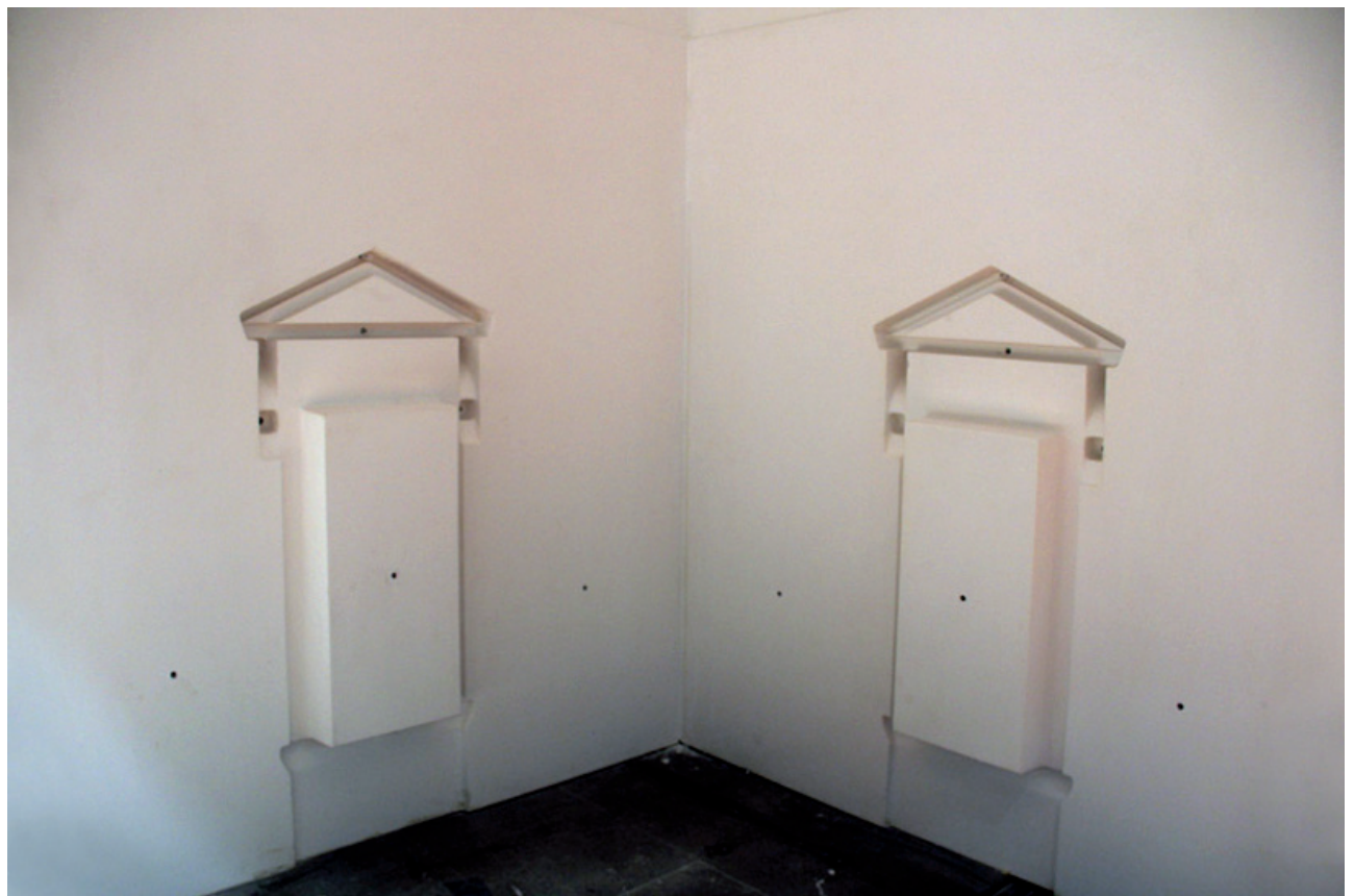
Fig.12c Interior of mould, windows added
