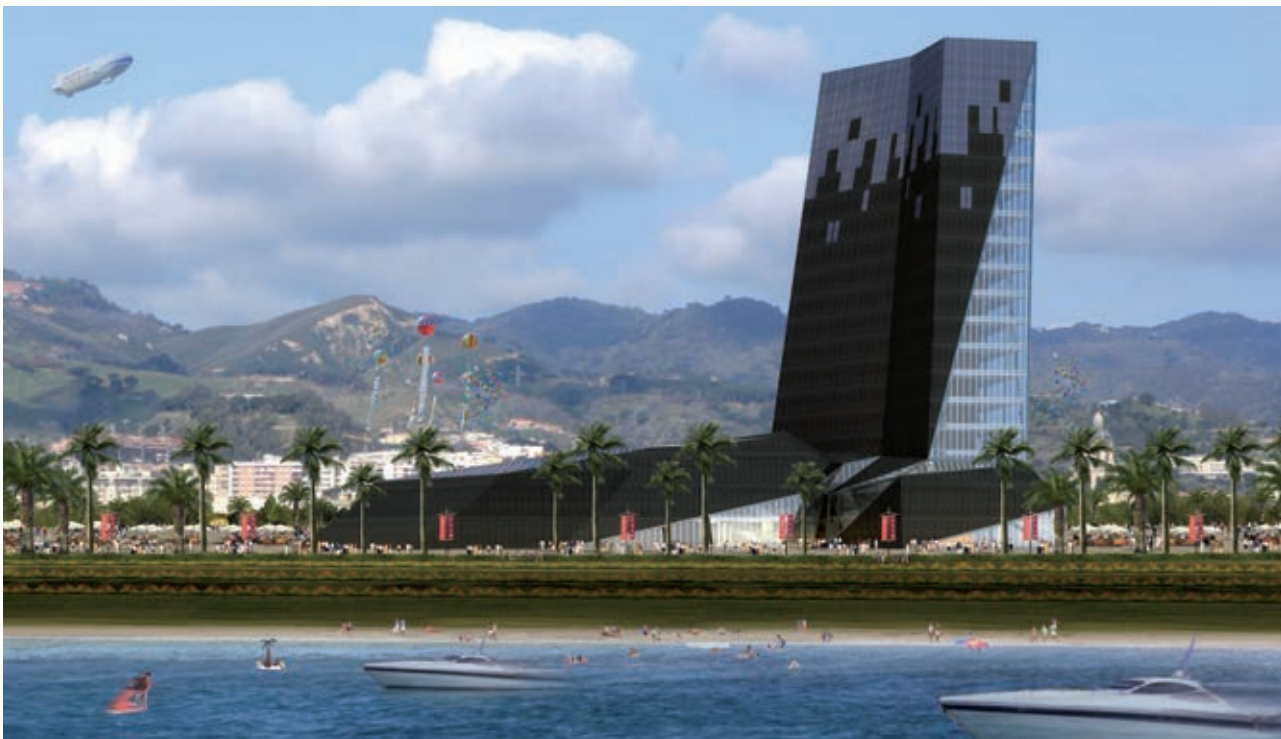
Fig. 08. Polycentre Tower from Sea showing Elevated Plaza
